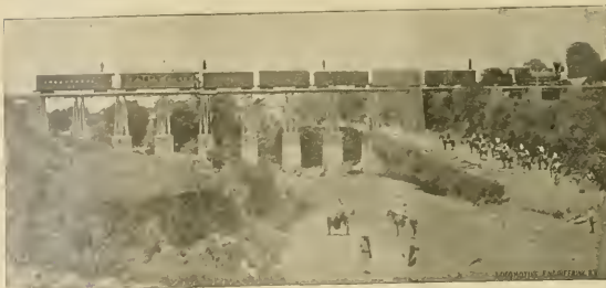
IDOACO BRIDGE, INTEROCCO RAILROAD, STATE OF MEXICO.
